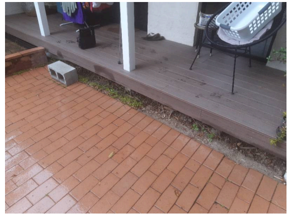
Example of timber decks at front of properties conceal weep holes.
